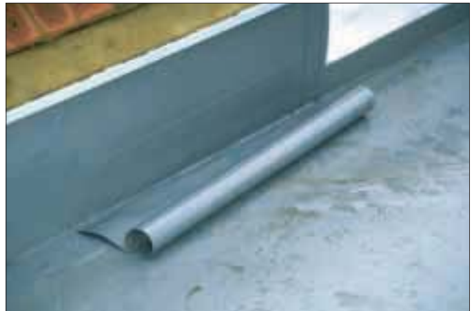
Fig. 3: Edge restraint with ALKORFLEX® metalsheet 81191.
