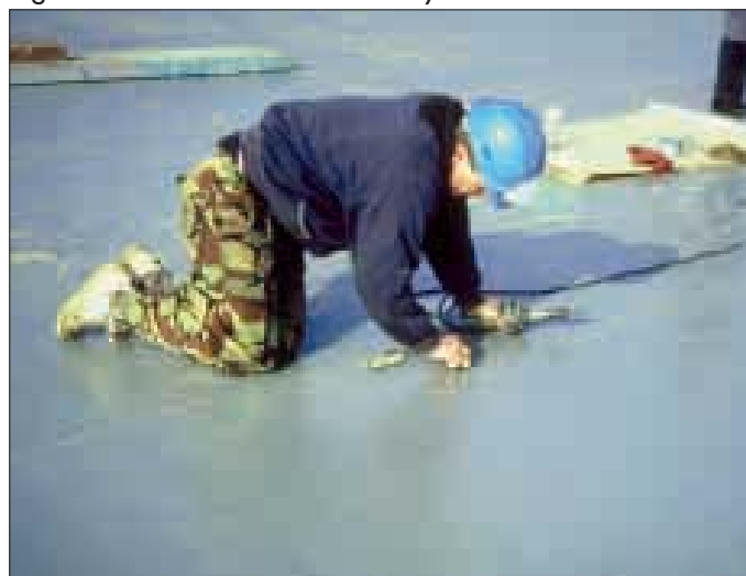
Fig. 2: Verification of weld security
