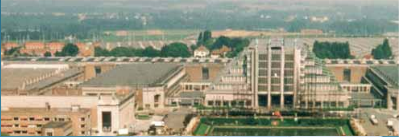
Project: Heyde Palace, Brussels, Belgium, 1985, 1990 Product: AquaPlan F (Mechanical Fastening, 70,000 sqm) Old waterproofing: Bitumen
