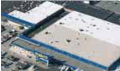
Project: Metro Etc. - Metro Group Product: AlkorPlan A (Adhered, 50,000 sqm) Old waterproofing: bitumen
