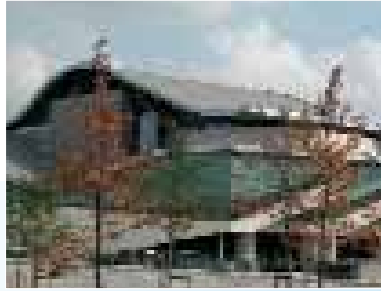
Project: Chassé Theatre Breeda, The Netherlands, 2002 Product: AlkorPlan® F (Mechanical fastening, 1,500 sqm) Old waterproofing: Synthetic
